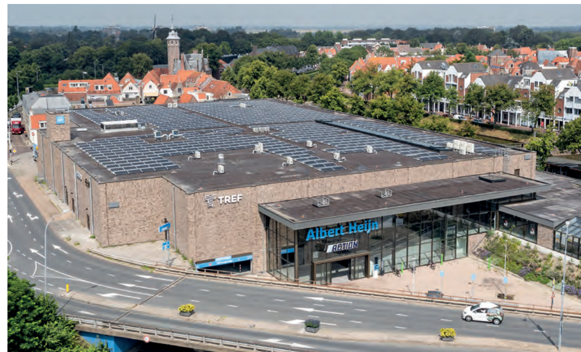
► Redevelopment of the convenience shopping centre TREF in Middelburg resulted in around a 60% decrease in energy consumption, from 345 kWh to 138 kWh per sq m, which is enough energy to power 300 homes every year
